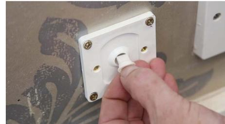
**7.** Insert one way valve in the centre of Back-Plate. Insert screws into plastic screw caps and fix Face-Plate to Back-Plate, clip on white screw cap covers.
