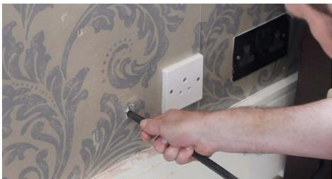
**5.** Fit a length of black tubing (enough to go through the wall) to the rear of the Back-Plate and insert tubing through wall.
