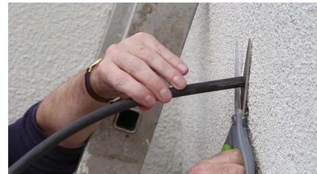
**8.** Externally: Cut off excess black tubing flush with the wall and attach elbow. Now run the Black Tubing towards the soil pipe using Elbows where required.
