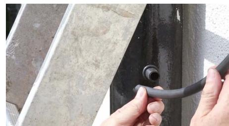
**10.** At soil pipe drill 20mm hole and fit rubber grommet. Cut Black Tubing so that it sits inside grommet approximately 20mm. **Installation is complete!**
