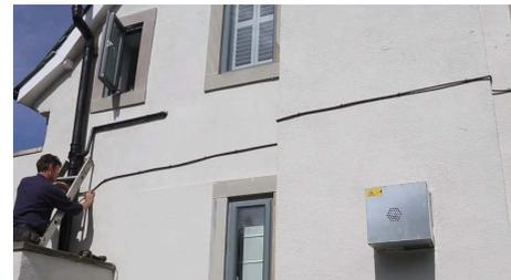
**9.** Run & fix Black Tubing along wall using "p" clips, screws & plugs. Be sure to create a good fall towards soil pipe.
