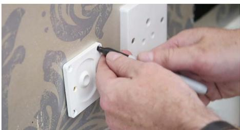
**4.** Place Back-Plate in position & make sure socket is level. When in position, mark out 4 x wall fixing screw locations.
