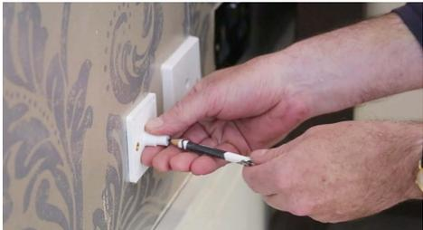
**2.** Choose a Wall Socket location that suits the user and bed position. Site as low as possible & mark out the centre of the Back-Plate.
