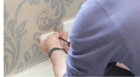
**6.** Position the Back-plate and fix with 4 x screws. Make sure that the screws are set below the front surface of the Back-Plate. Do not over tighten as this will distort the shape of the Back-Plate.
