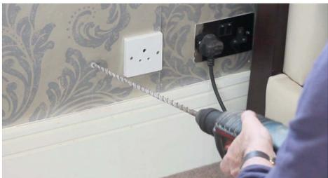
**3.** Drill a 14mm hole with adequate fall (approx 6 degrees) away from the socket. (use a 10mm bit to drill a pilot hole first if available).
